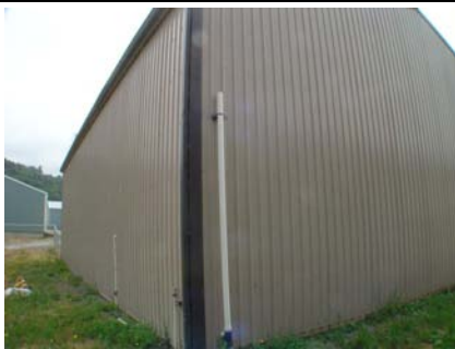
NW General Site
