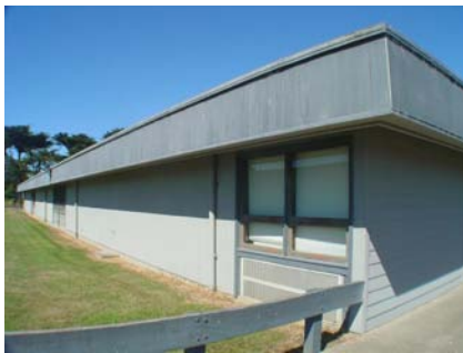
SW General Site
