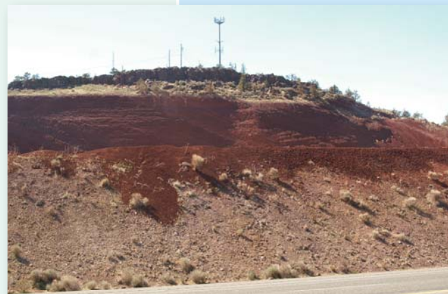
Cinder Butte Rock Products has established a berm around the perimeter of the pit that effectively screens the processing and stockpile areas, and also acts as a noise barrier.
